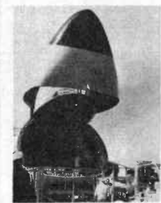
BIG MOUTH . . . A U. S. Air Force C-g Galaxy Visor nose, recently patented, opens wide to expose mammoth transport's 19-by-13½-foot cargo compartment stretching 121 feet forward and aft loading ramps.
